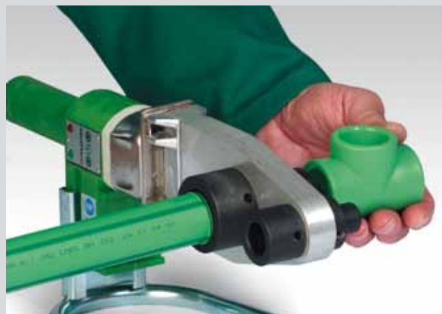
Heating-up of pipe and fitting
