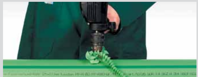
Drilling through the pipe wall
