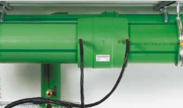
Adjust the socket diameter on the welding device. Start and control welding process. Keep the cooling time. Finished!
